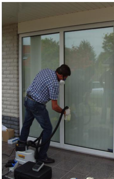
Fig. 1 Spraying the self-cleaning coating on a window (Company 1)
