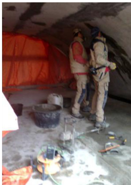
Fig. 2 Manual concrete repair at the underside of a bridge (Company 2, location 1)
