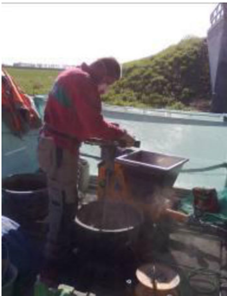
Fig. 3 Mixing concrete repair mortar (Company 2, location 2)
